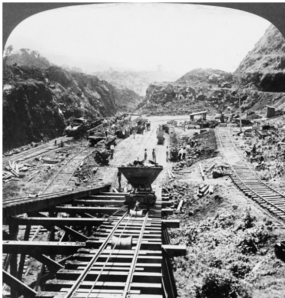
Above: The construction of the Panama Canal.
